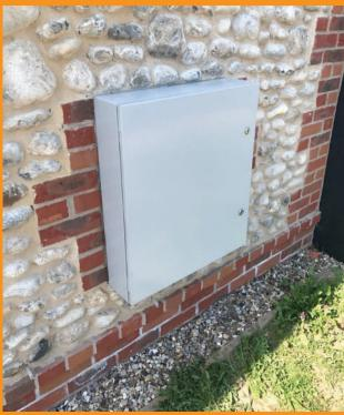
Waterproof Flood Cabinets can simply be retrofitted over the existing metre box to ensure a passive, 'automatic' flood protection solution.
