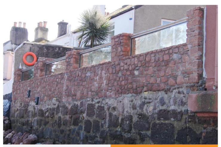
Our Glass Flood Walls are designed as a permanent feature, thus providing continuous flood protection and requiring no operation. However, the modular nature of the system allows for individual glass panels to be removed or replaced if required, whilst not having to demount or replace the entire span.
