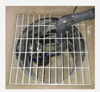
The submersible pump system is installed below ground to a bespoke sump. The pump has an integrated float switch which enables it to automatically switch itself on in the event of rising water, pumping water out and away from the premises.
