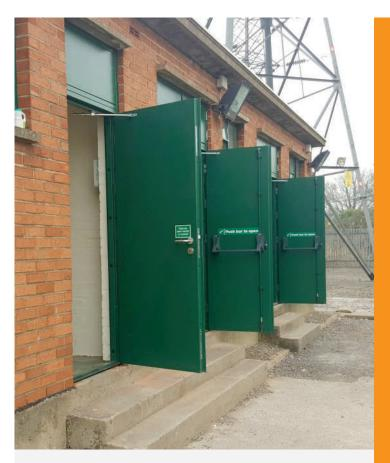
Steel Fire & Flood Doors ensure robust protection against both flood and fire risk. The flood doors are designed and manufactured to the highest specification with unique seal mechanisms and hardware, resulting in flood protection to full door height.
