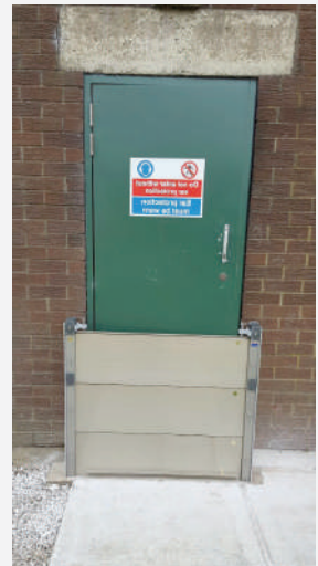
Fire Exit door
